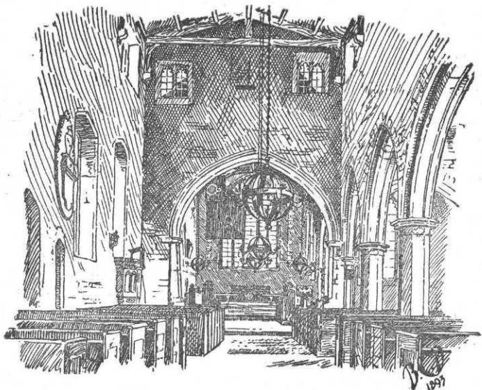
HAWKESBURY CHURCH: INTERIOR, LOOKING EAST.
