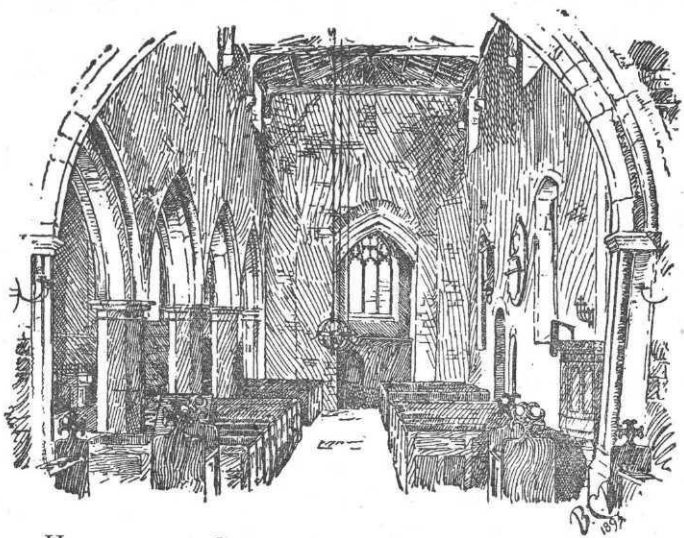
HAWKESBURY CHURCH: INTERIOR, LOOKING WEST.
